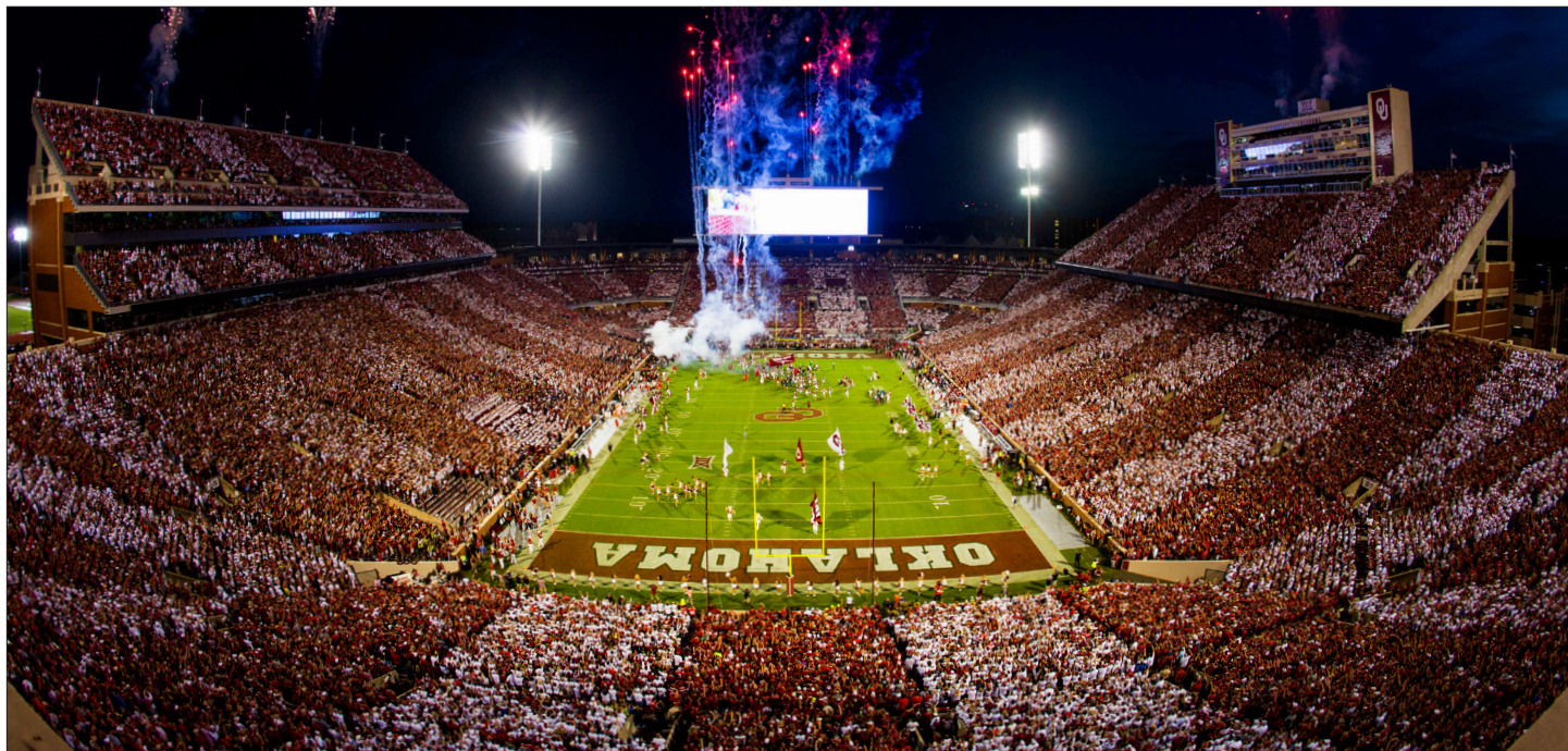
OU's $160 million stadium renovation and modernization project bowled in the south end of the facility and added premium seating and a 62-foot-by-38-foot video board.
